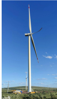
Wind power tower weld inspection
