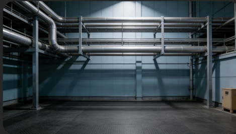
Buildings & Utility Tunnels
